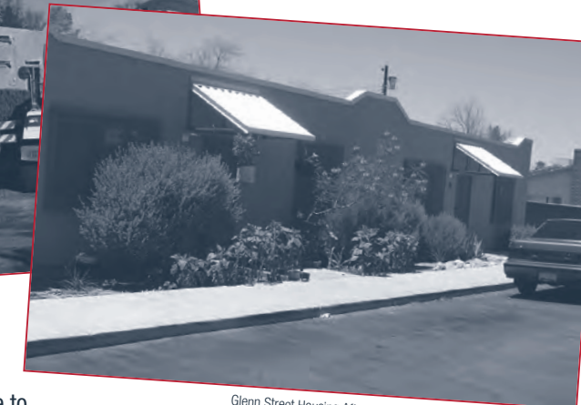
Glenn Street Housing After
